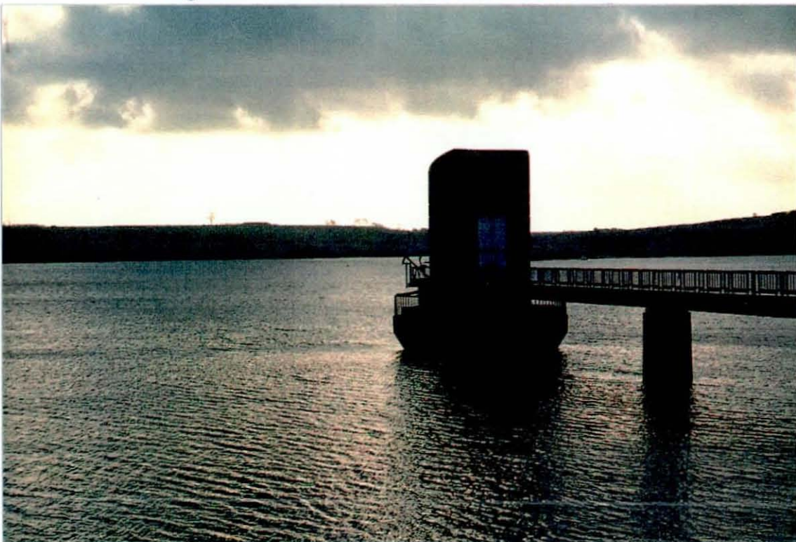
Fig.5.3/1 Foremark Reservoir and Draw Tower
