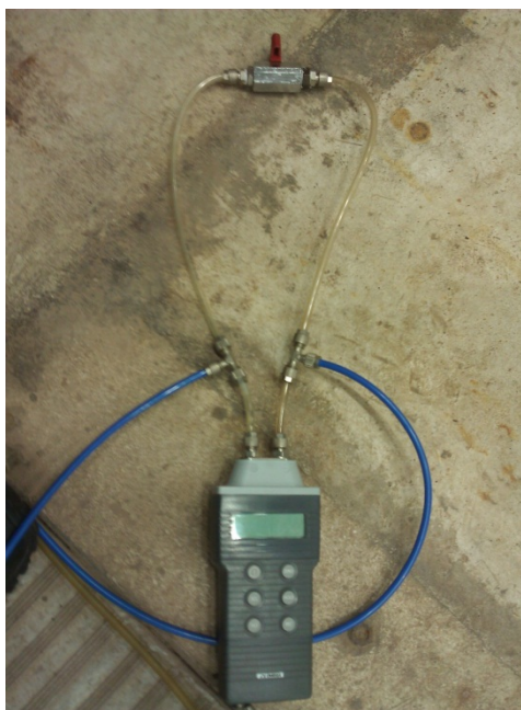
Figure 70 - Pressure transducer and air removal loop
