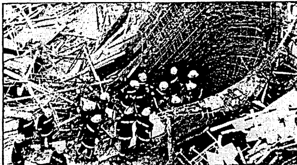
Firemen search the wreckage of the collapsed canopy.
