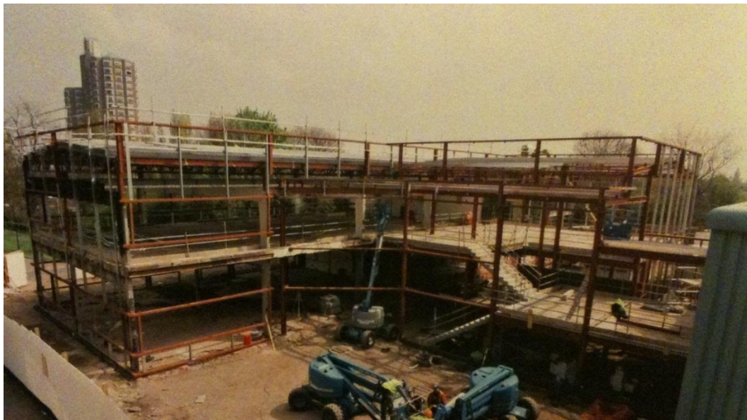
Figure 7-7: Structural adaptation to original structure
