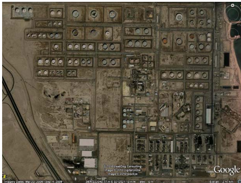
Figure 4.6: KNPC's MAB Refinery
