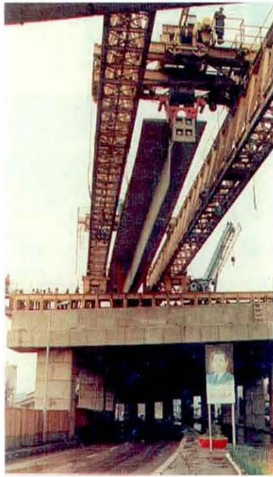
Figure 3.36: Launching Trusses moving transversely to erect precast beams (The Arab Contractors, 1995)
