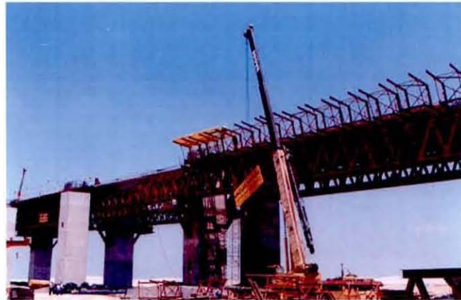
Figure 3.25: The system lifted into position using cranes (The Arab Contractors, 2000)
