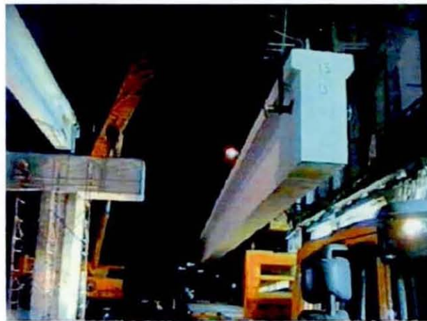
Figure 3.40: Precast beams erected using cranes (The Arab Contractors, 2004)
