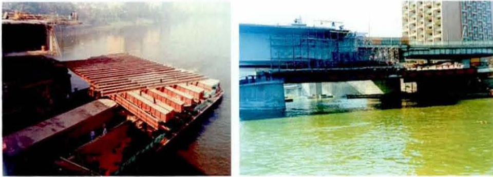
Figure 3.45: Creating an elevated platform and erecting falsework (The Arab Contractors, 2004)
