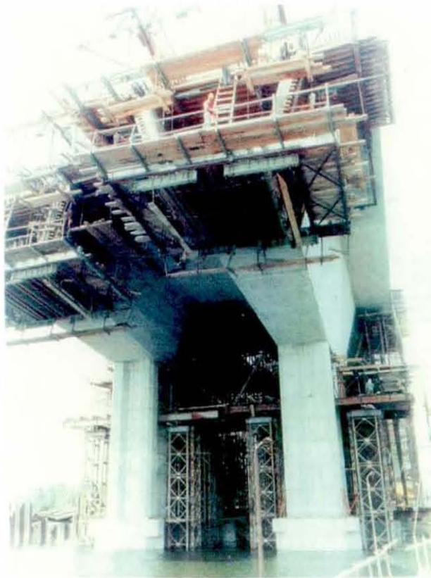
Figure 3.12: Vertical application of Bailey panels (The Arab Contractors, 1991)
