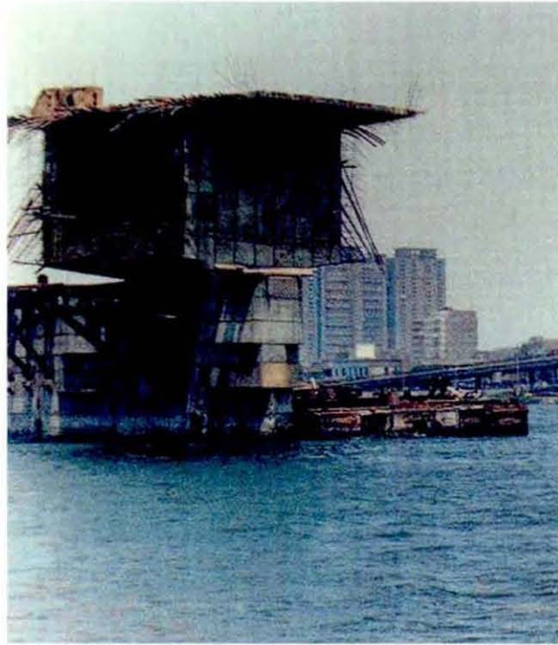
Figure 3.18: Finished Stump Using Steel Brackets (The Arab Contractors, 1996a)
