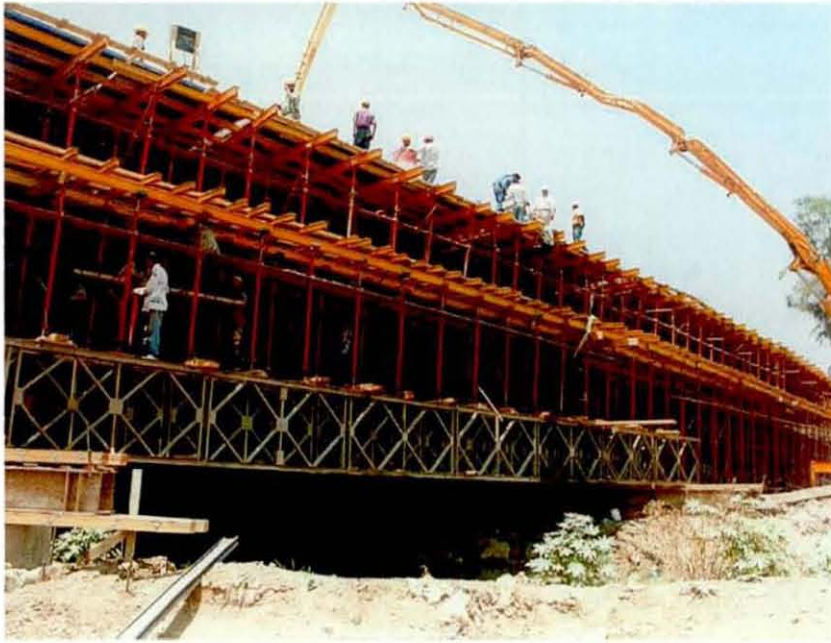
Figure 3.11: Horizontal application of Bailey panels (The Arab Contractors, 2004)
