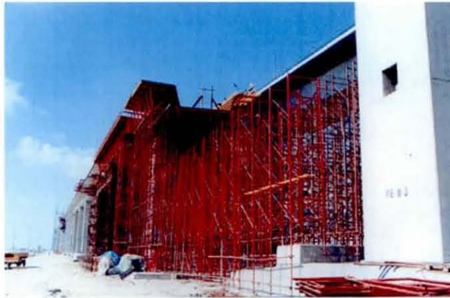
Figure 3.9: Falsework components during striking (The Arab Contractors, 2000)
