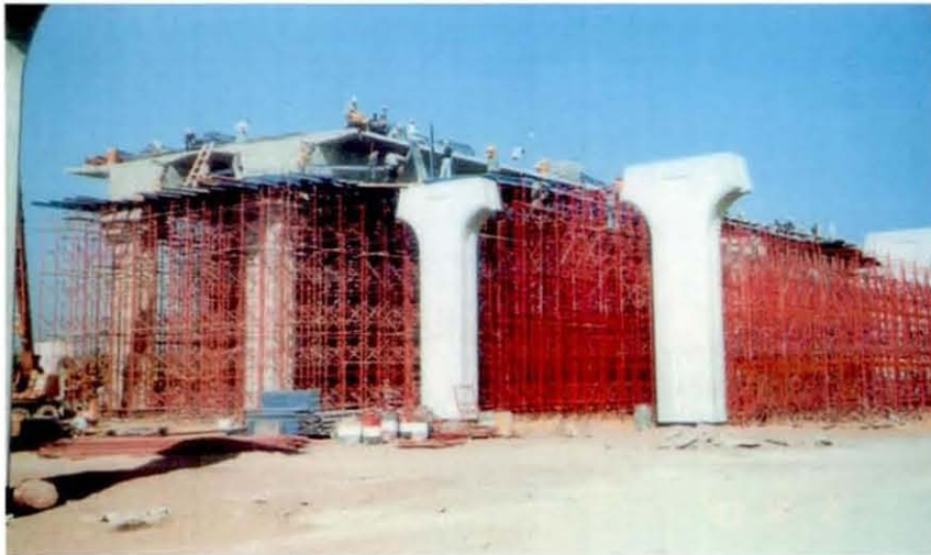
Figure 3.8: ACROW system used in Construction (ACROW Misr, 1995)
