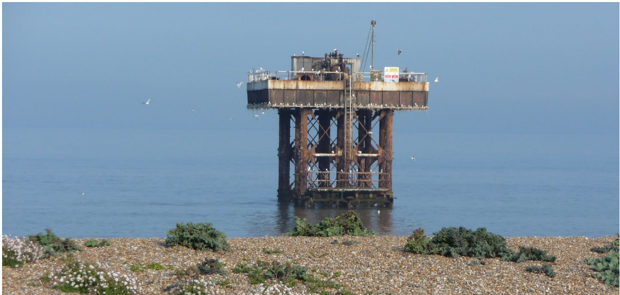
Plate 2 The (decommissioning) Sizewell A station (Magnox) cooling water outfall headworks
