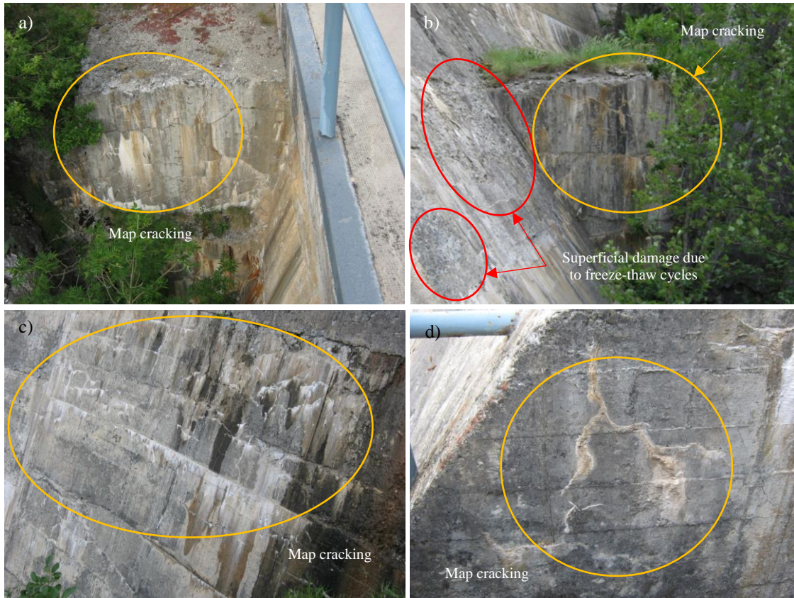
Figure 11. Map cracking localized in specific areas of the dam: a) block beside the right abutment, b) block beside the left abutment, c) downstream face and d) entrance to the upper gallery.
