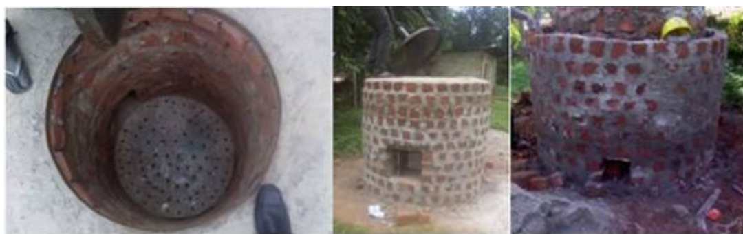
Figure 2. Masonry kiln design
