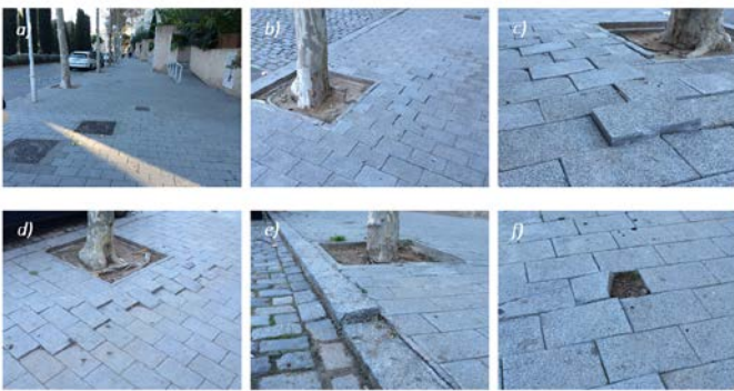
674 Figure 12. Different images of distresses in Carrer Moscou
