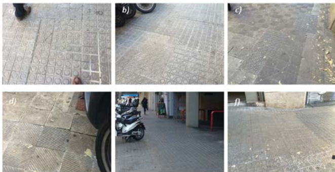
Figure 10. Different images of distresses in Carrer Bruc
