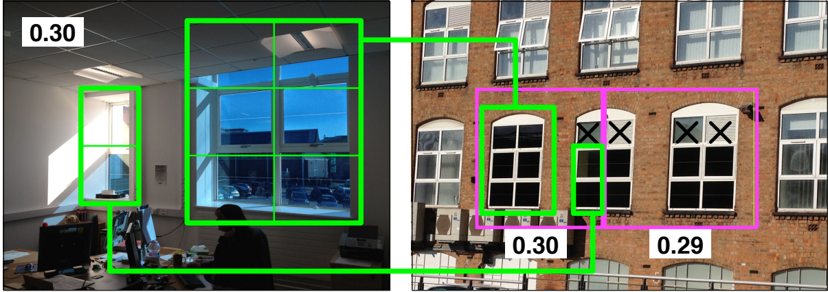
Figure 6: Photograph of Room 0.30 and the external facade.
