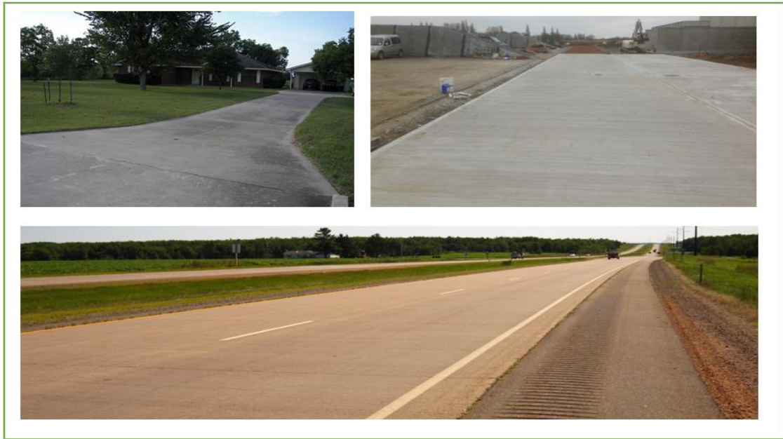
Figure 5-10 Concrete road images.
