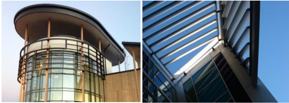
Figures A.8- Examples of Applied External Solar Shading Devices- Solinear (2013a) and Solinear (2013b)
