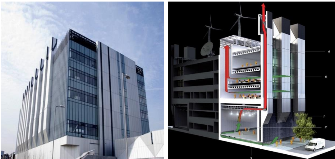
Figure A.2- Harlequin 1 building, London, UK (Michler, A, 2010) and Natural Ventilation Method for Studios (Building, 2014)
