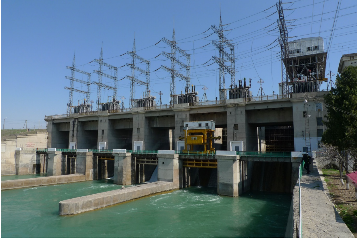
Figure 3.6: Kayrakkum hydropower plant (Michael Friedhoff)
