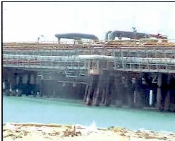
Figure 6.9 TPI factory and the harbour
