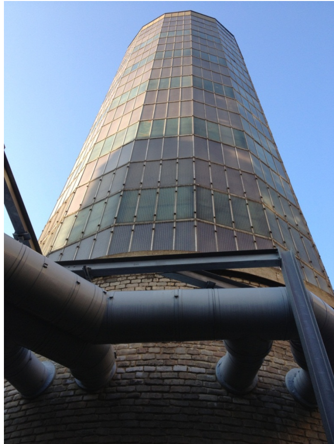
Figure 22. The thermal storage tower has architectural appeal
