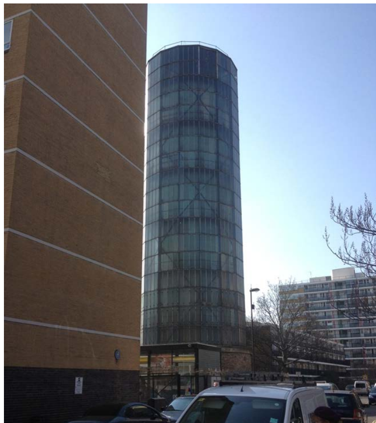
Figure 19. The thermal store at Pimlico District Heating Undertaking
