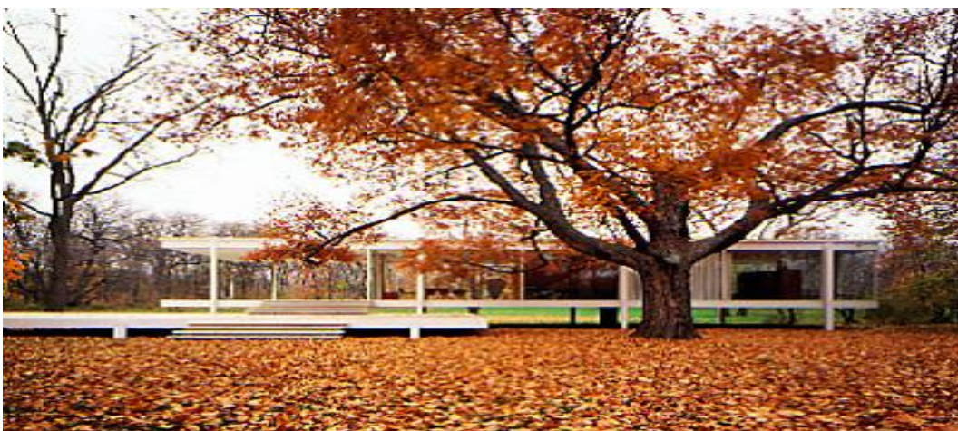
Figure 2.2 Farnsworth House, developed by architects Mies Van er Rohe (Rose, 2007)
