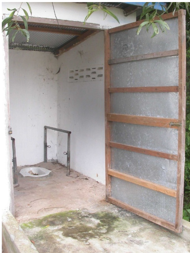
Figure 3. Latrine with handrails and wide door
