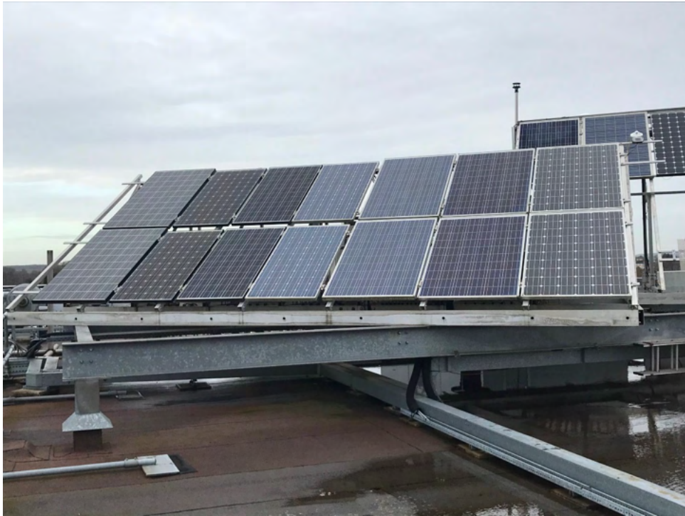
Figure 5-1 Installation of the PV modules on the roof.
