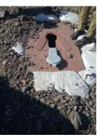
Figure 3: A lined pit with slab.
