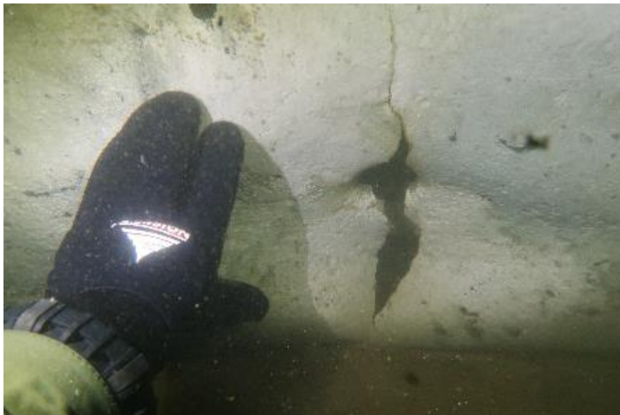
Figure 2: Mine November - Pluton Injection Point and Minor Overpressure Damage
