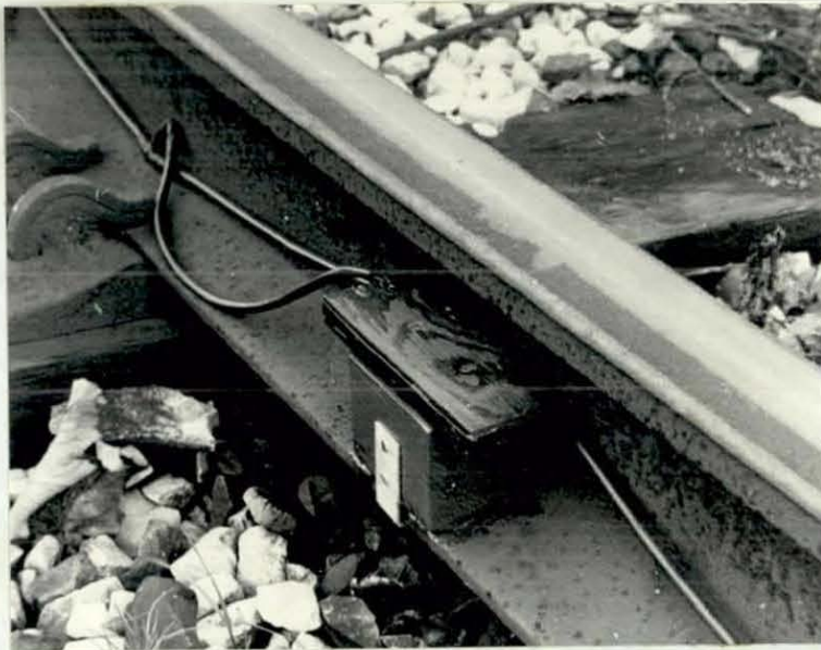
Fig. 112. Photograph of Telegram Coil and Fixing.
