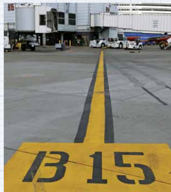
The simplest way to guide an aircraft on to its stand is using markings painted on the tarmac/concrete surface. But these alone do not tell a pilot exactly when to stop so that he is aligned with the airbridge and ground equipment. (KEY Collection)
