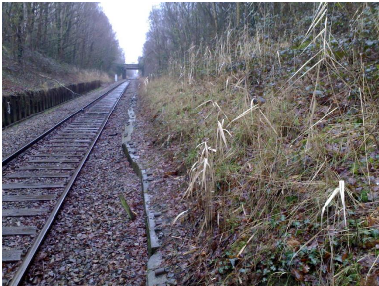
Figure 4.15. Photograph of the toe of the Players Crescent slope showing distorted concrete cable trough and toe bulging
