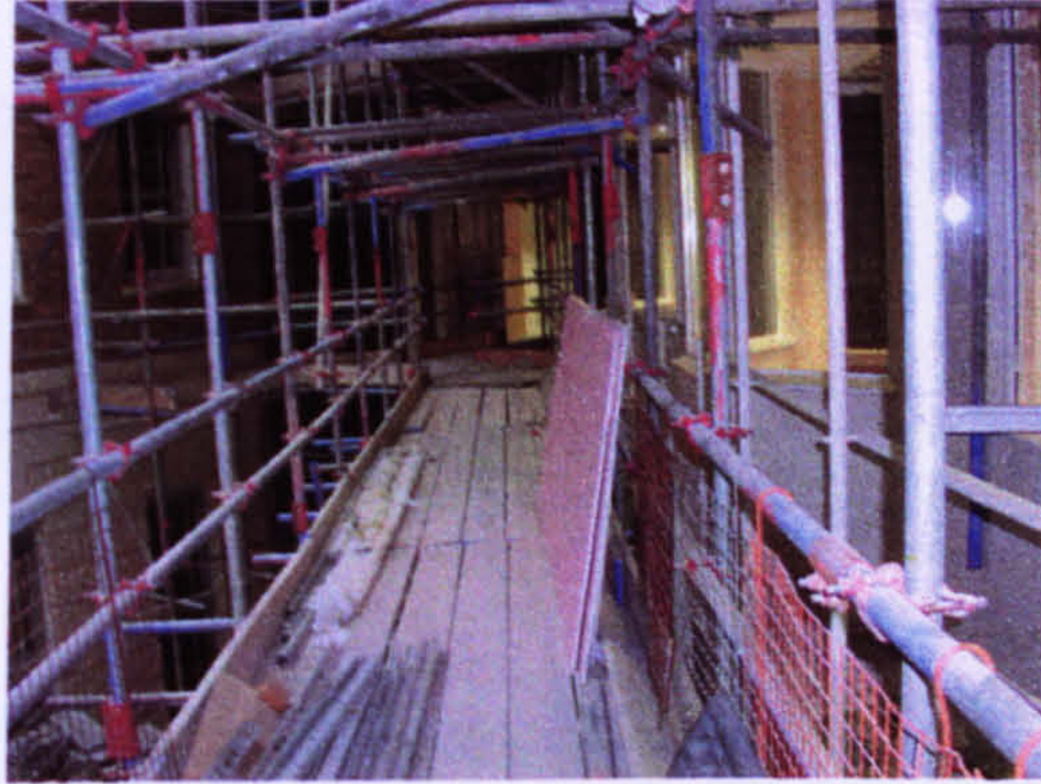
Clips stick out into the walkway Plasterboard 8' x 4'
