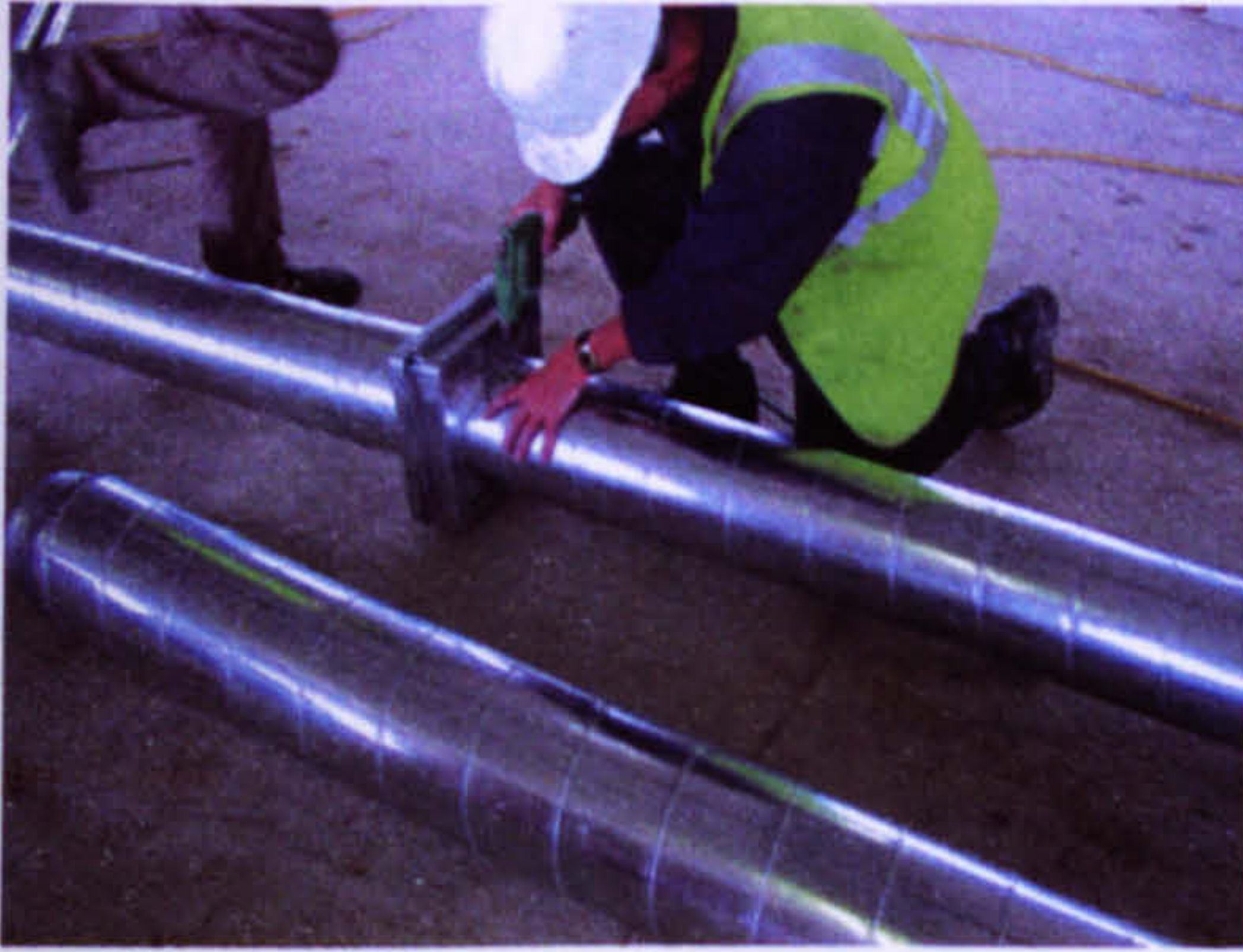
Staged hole drilling exercise
