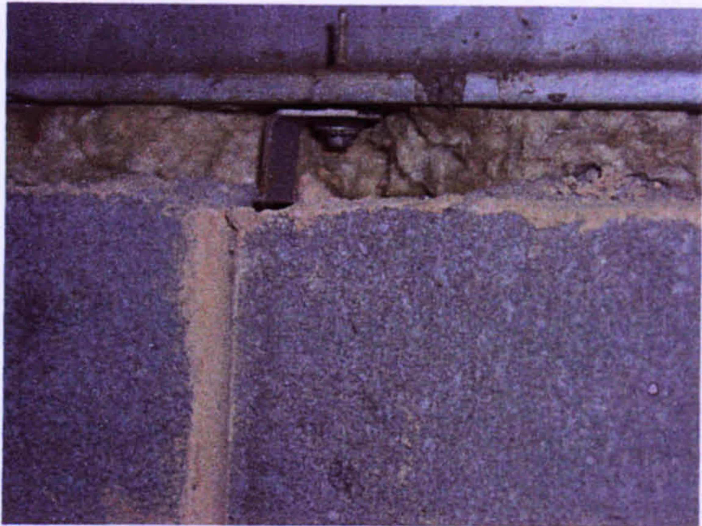
The rivet through the steel and securing block
