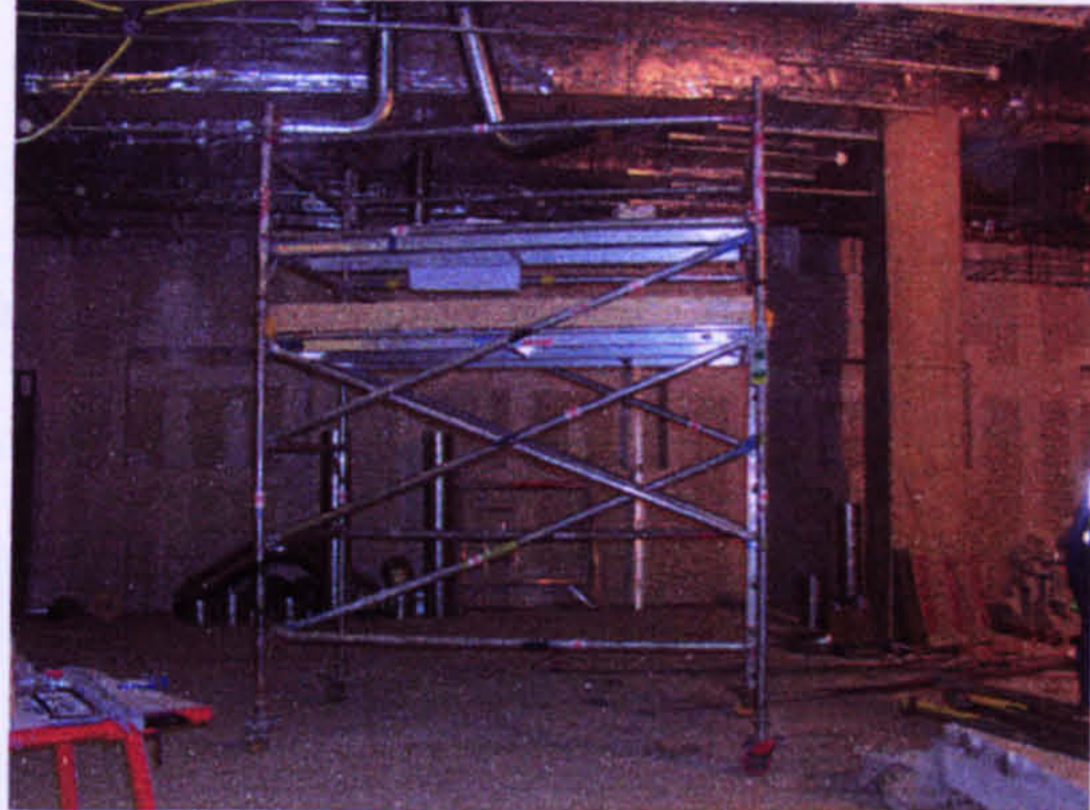
Typical boards that were tripped on except that the one in question had another rise on it taking it up to 4m high.
