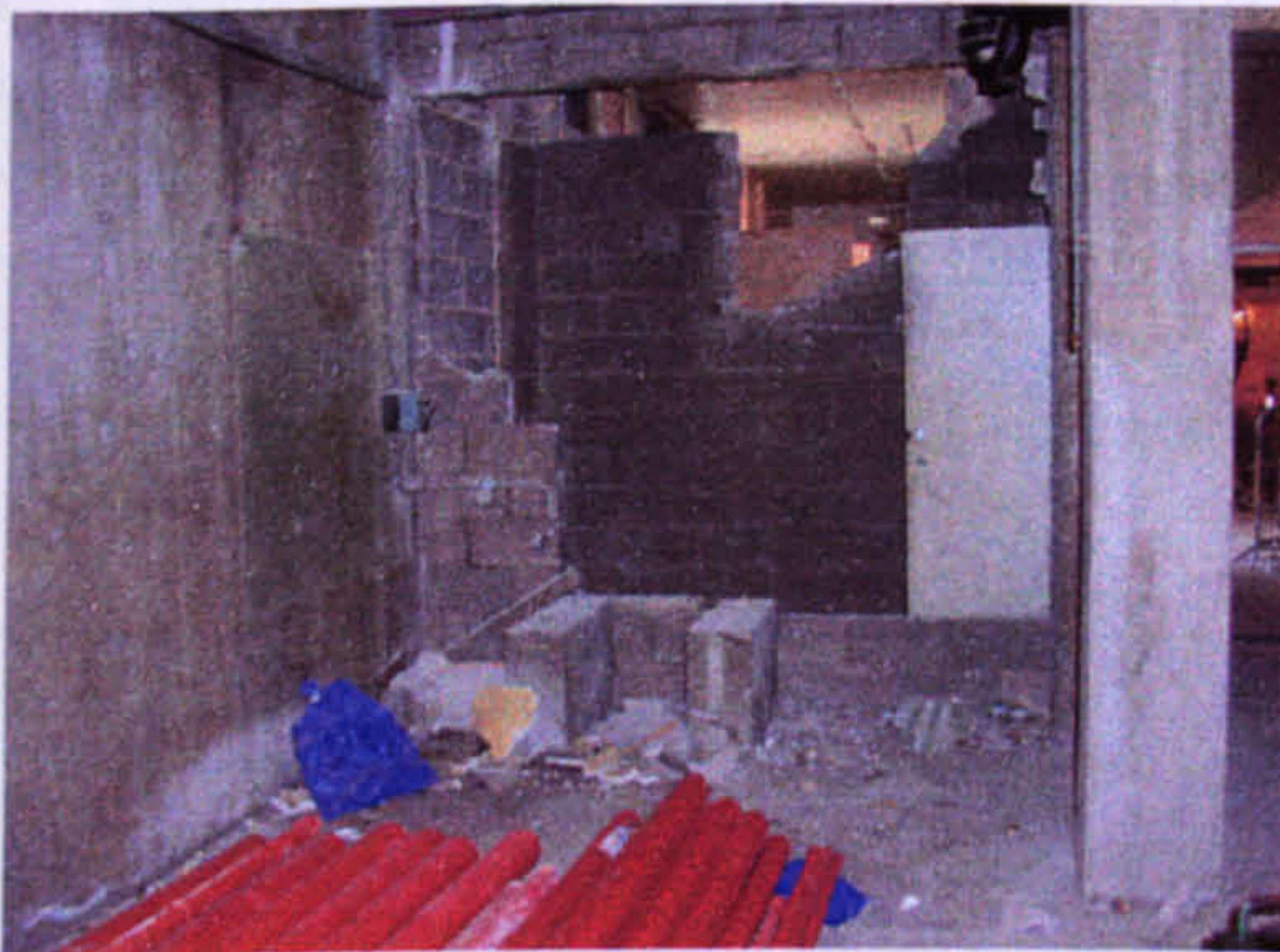
Hole left by duct + structure IP was squashed against
