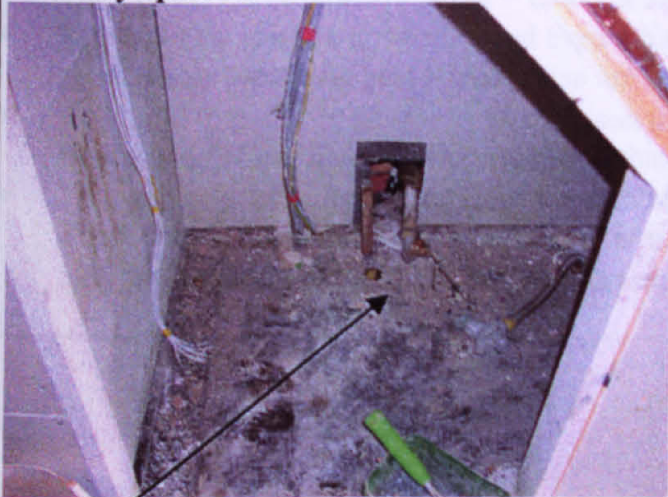
Hole where old gas pipe was cut off. New pipes now in position
