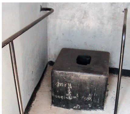
Figure 8. Raised toilet seat with rails fixed to wall and floor 6
