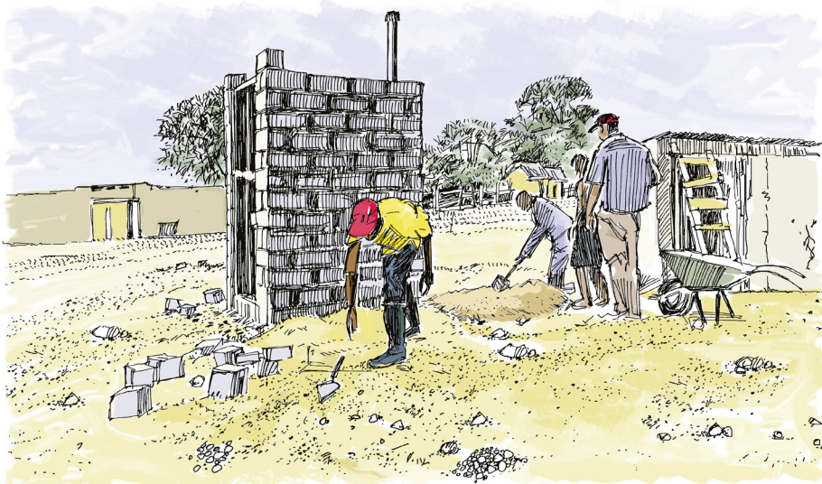
Figure 6. A VIP latrine under construction
