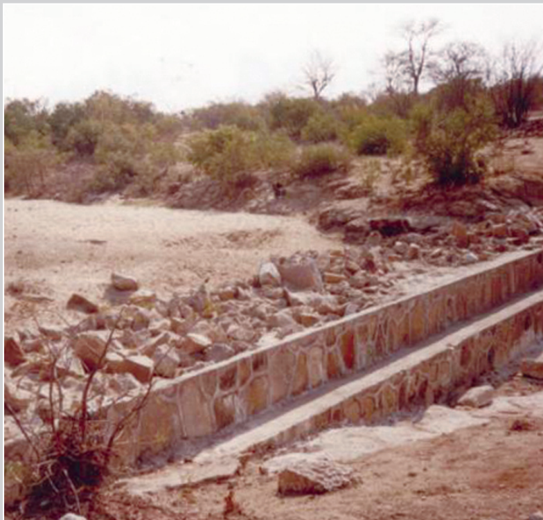
Photograph 4.10. Mkayi Wokhoza sand dam under construction
