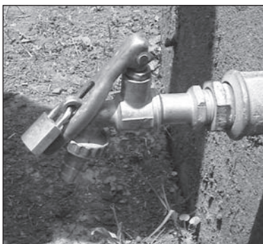
Figure 9.102. The tap can be padlocked.
