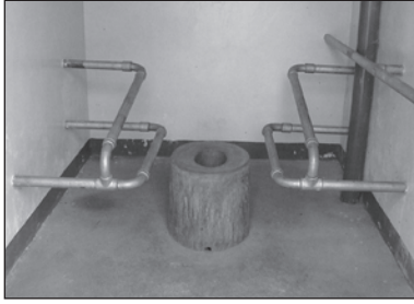
Figure 9.124. Raised toilet seat with handrails for support.
