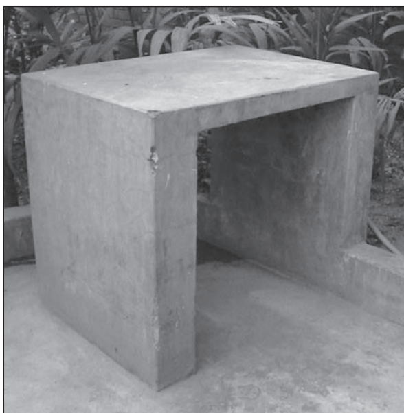
Figure 6.83. Concrete slab for washing clothes. (Case-study 9.3, page 166)
