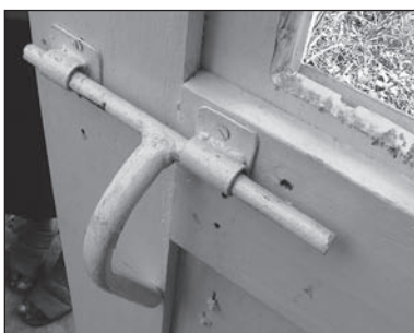
Figure 9.123. Large slide bolt for easy grip.
