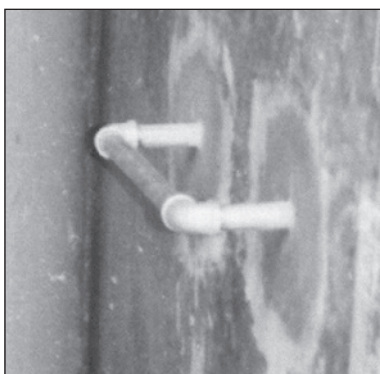
Figure 9.144. Handrail cemented to the wall.
