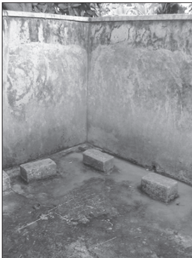
Figure 9.121. Fixed concrete sitting blocks for bathing.
