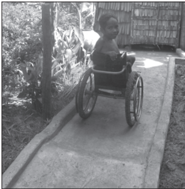
Figure 9.68. Concrete ramp leading to bathing area.
