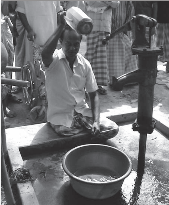
Figure 6.48. Low concrete sitting platform. (Case-study 9.2, page 161)
