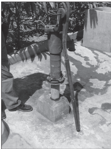
Figure 9.14. Water drains away from the apron.
