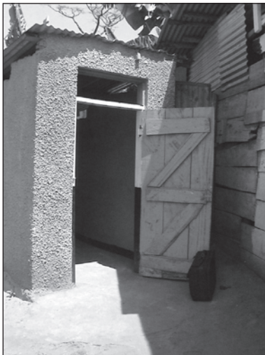
Figure 9.118. Door with a two-way hinge.
