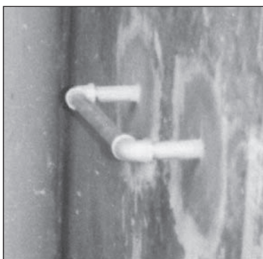
Figure 9.144. Handrail cemented to the wall.
