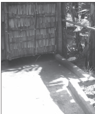
Figure 9.71. Flat platform in front of toilet door.
