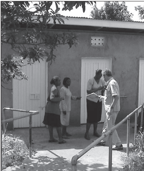
Figure 5.10. Wide concrete ramp with handrails both sides.
