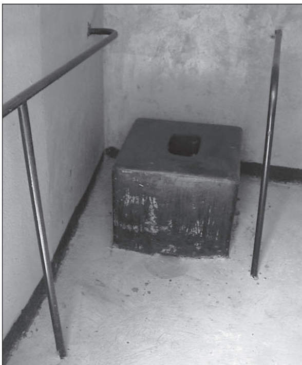
Figure 7.7. Painted rail fixed to floor and walls.
