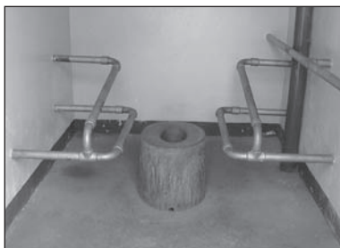
Figure 9.124. Raised toilet seat with handrails for support.
