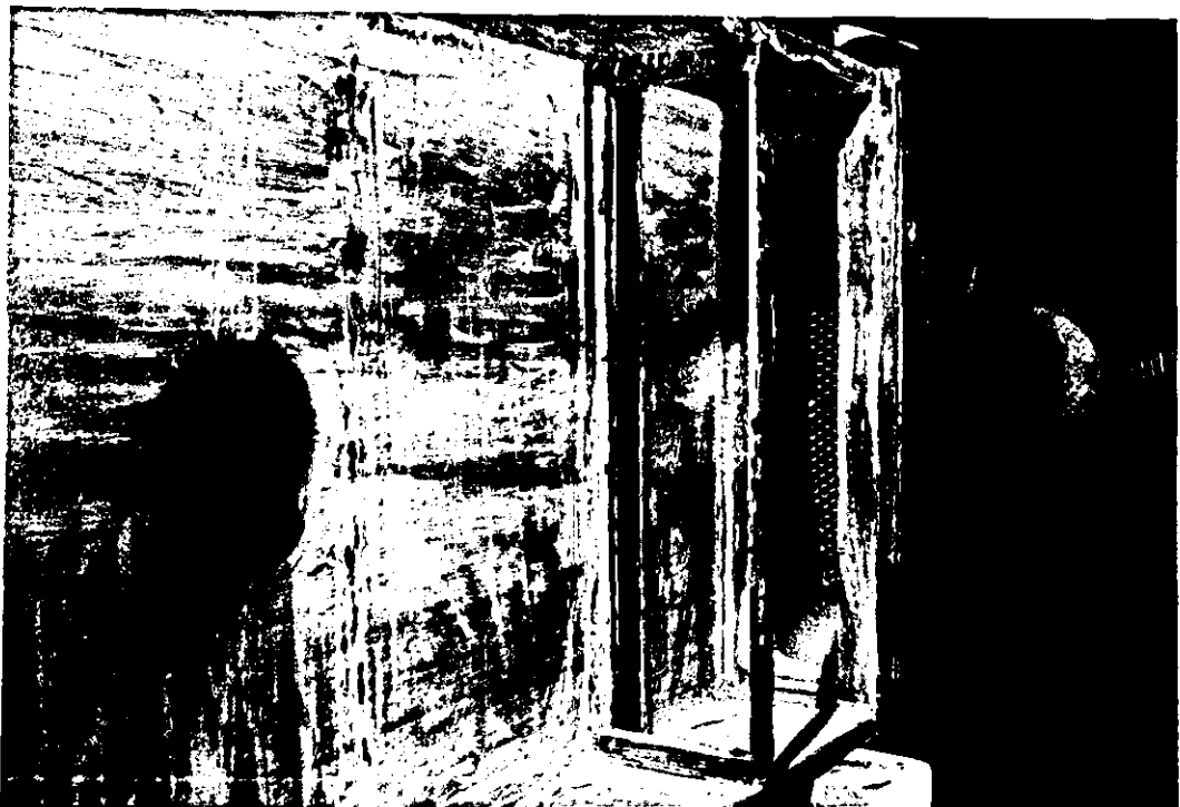
FIGURE 4.15: Filter box with deeppleat filter support frame
