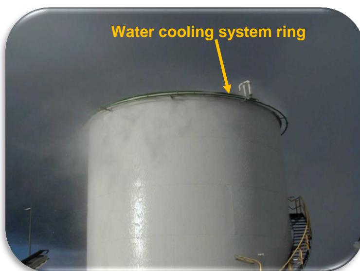
Figure 5.1: A water cooling system was applied, in order to cool a storage tank. The type used consisted of a fixed ring installed around the top of the tank wall ( www.saval.be )
