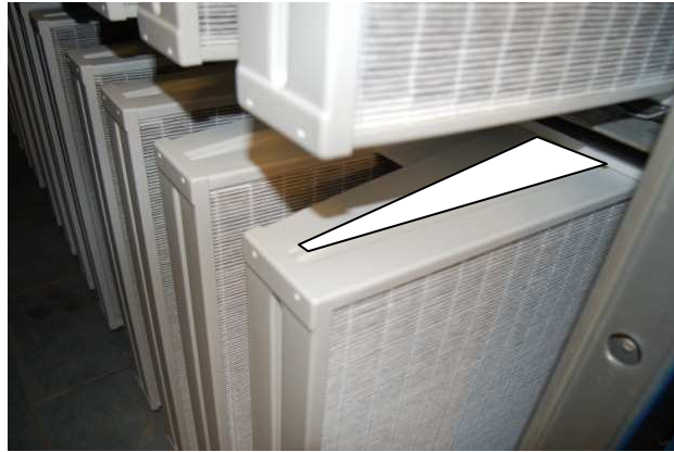
Figure 5.3: Top view of the pleated filter suggested to be replaced with pleated medium.
