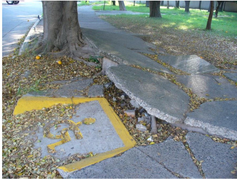
Figure 5.11 Example of a pavement in bad conditions due to growth of roots tree
