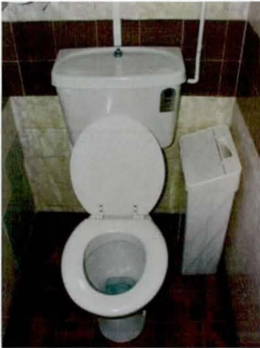
Figure 6.8: Toilet with IR flush
