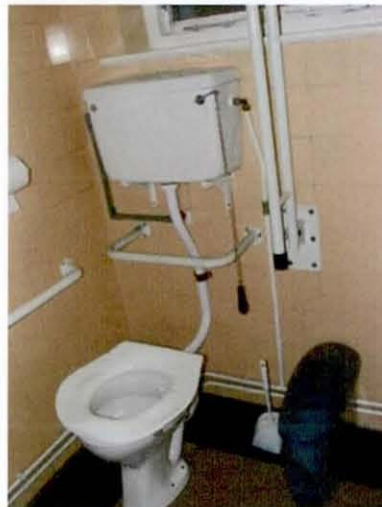
Figure 6.11: Toilet with chain flush
