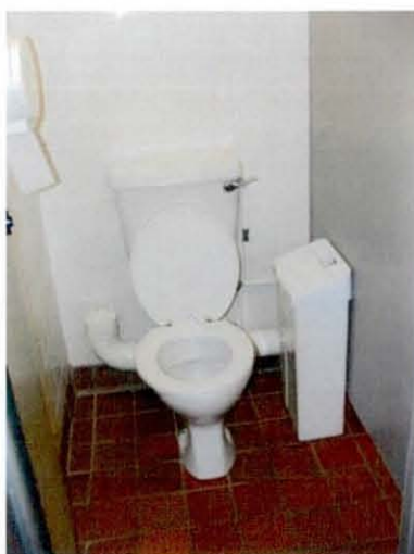
Figure 6.16: Sanitary waste unit located between the dividing wall and toilet
