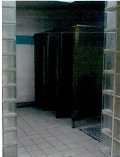
Figure 5.3: Cubicle dividers and doors with gaps at the top and bottom
