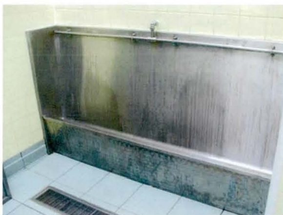
Figure 5.12: Stainless steel trough urinal
