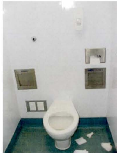
Figure 6.22: In wall sanitary waste unit
