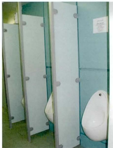
Figure 5.14: Full-length dividing screens at urinals
