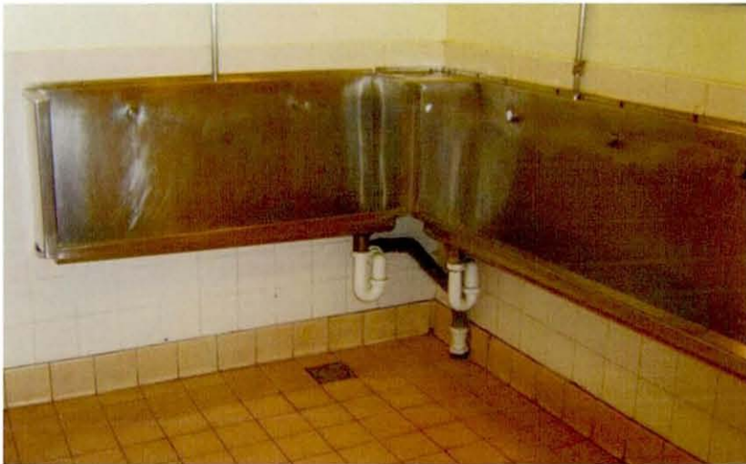
Figure 2.26: Stainless steel trough urinal
