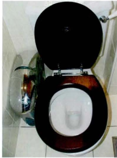
Figure 2.30: Sanitary waste unit between the toilet and wall
