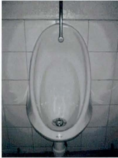
Figure 2.25: Individual vitreous ceramic urinal
