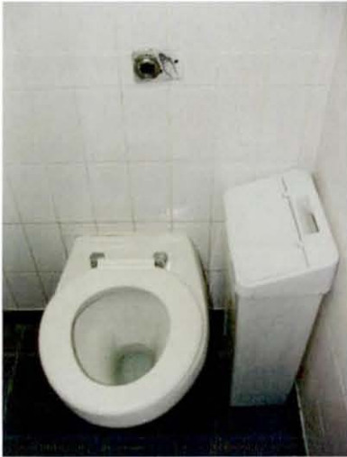
Figure 6.19: Hand operated sanitary waste unit
