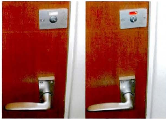
Figure 6.2: Empty cubicle; confusing vacant and engaged signs on lock
