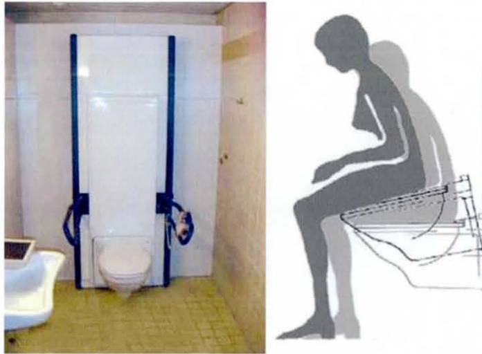
Figure 2.20: FRR adjustable toilets, height and tilt (Panek et al. , 2005)
