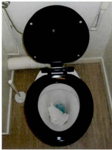
Figure 6.3: Toilet paper placed in bowl to reduce splash back and scarring
