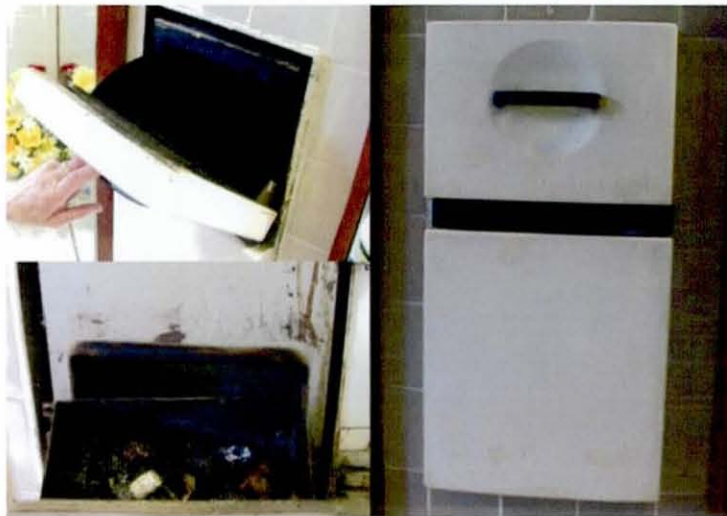
Figure 6.17: Sanitary waste incinerator
