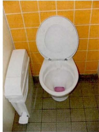
Figure 6.20: Pedal, foot, operated sanitary waste unit
