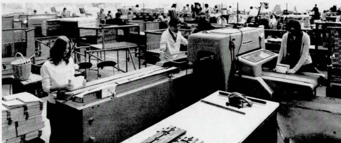
Figure 11: Wohlenberg three-knife trimmer in the bindery of Wills and Hepworth Ltd.
