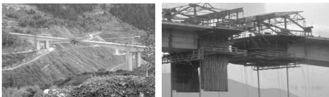
Figure 2. Views of under construction Metsovo ravine bridge a) General view b) key of central span.
