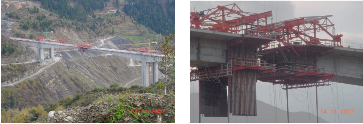
Figure 3: Views of under construction Metsovo ravine bridge, (a) General view, (b) key of central span.
