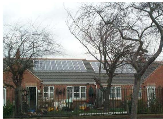
**Figure 2:** The shaded PV system (the array on the left) with the surrounding trees and pitched roof
