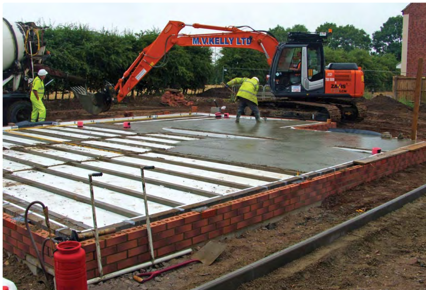
Figure 1: Placement of self-compacting concrete into residential house slab.
