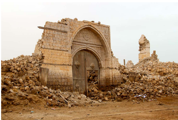
Figure 2. Deterioration of Suakin's historic coral block buildings
