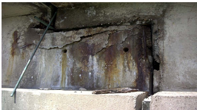
Figure 8. Chloride induced corrosion deterioration of a bridge half-joint
