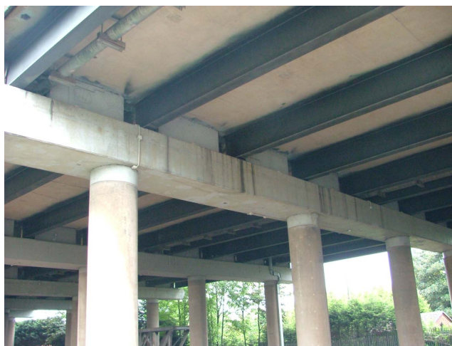
Figure 6. The first operational ICCP system on the MLMV installed in 1990 as seen on 14/03/2012
