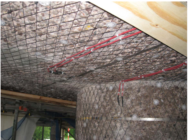
Figure 7. A MMO/Ti mesh fixed to a concrete beam prior to the application of the cementitious overlay
