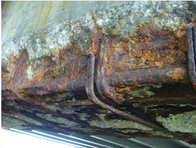
Figure 1. Typical chloride-induced corrosion damage to a reinforced-concrete structure
