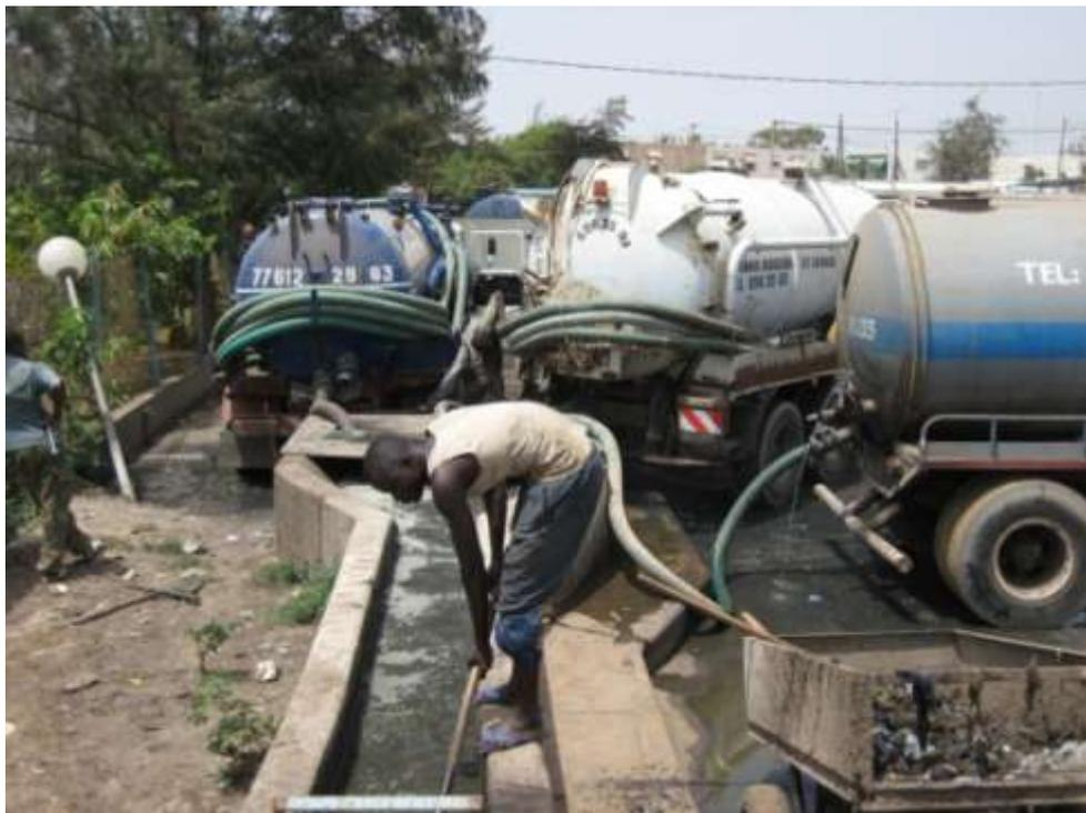
Figure 10-20: FS treatment centre Cambarène Dakar, worker manually removing foreign material from grate (taken by author 2008 Dakar)
