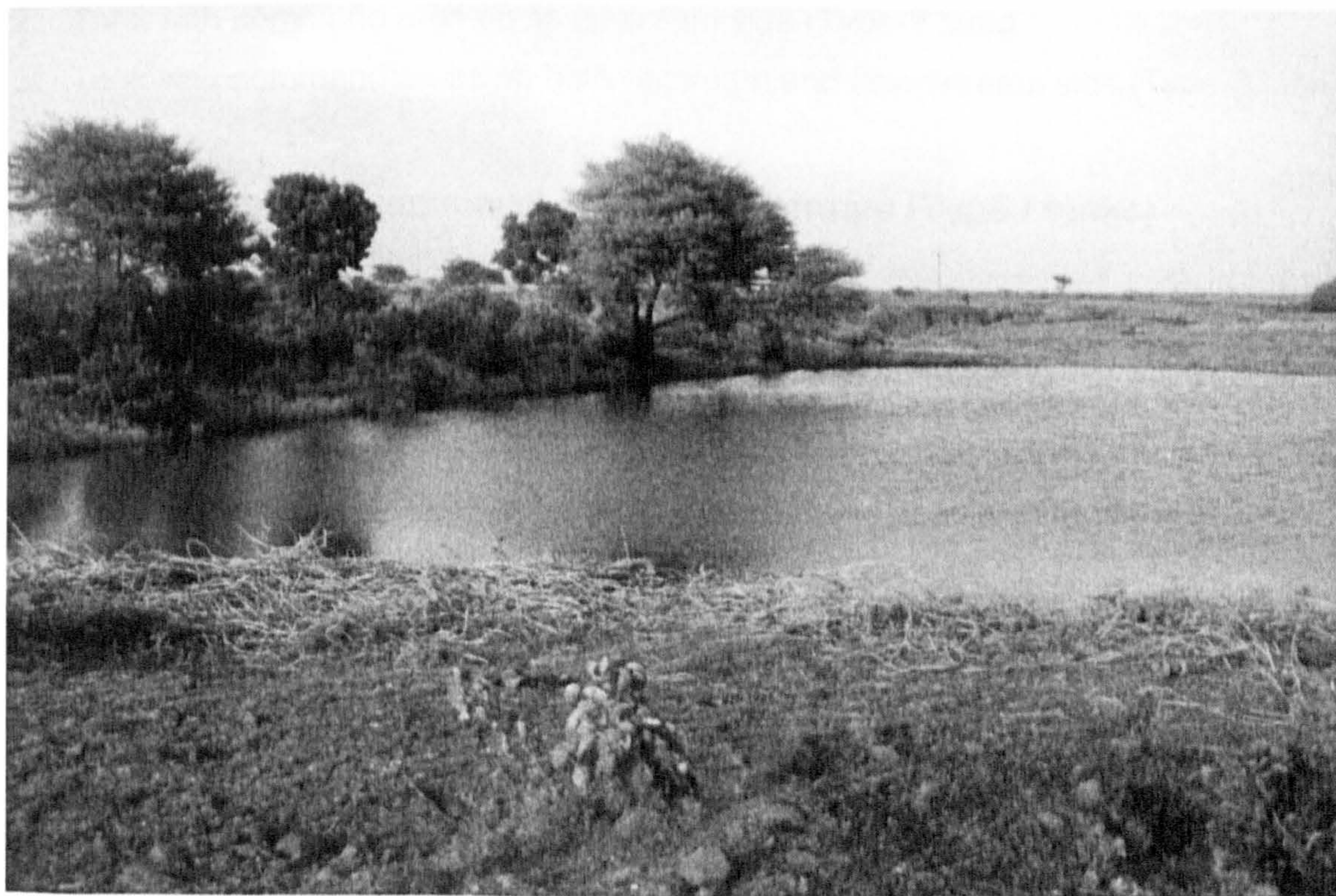
Figure 4.2 An excavated tank (farm pond) for irrigation (Source: MPKV, 2001)
