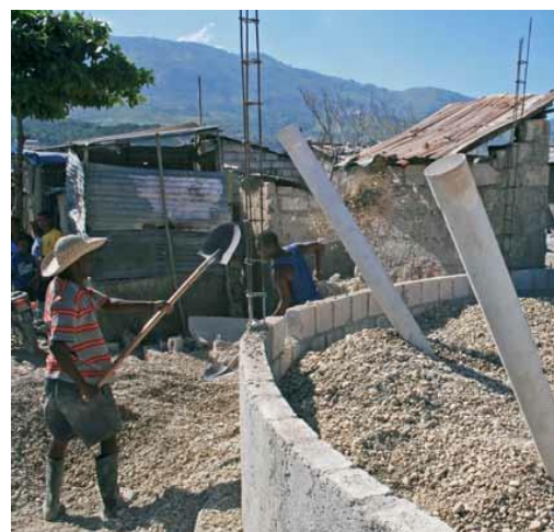
Figure 5.11 Household owned latrines being constructed within existing neighbourhoods as a part of Oxfam's long-term sanitation strategy. [Source: Oxfam 2012]
