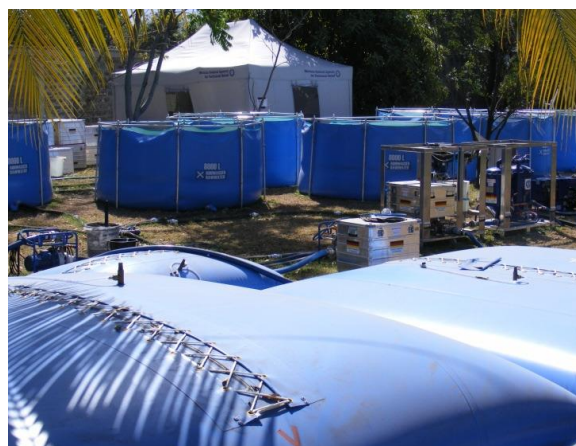
Figure 5.9 Water storage through water bladders used to supply the vast quantities of treated water to the thousands of IDP camps in PaP. [Source: DINEPA 2012]
