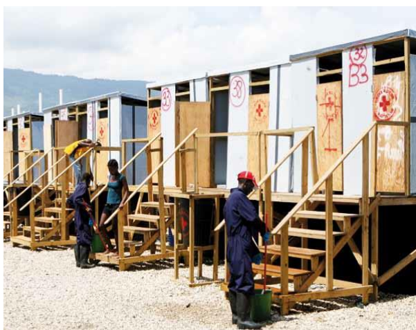
Figure 5.10 Some of the thousands of above ground latrines that were constructed throughout the IDP camps in PaP. [Source: IFRC 2010]
