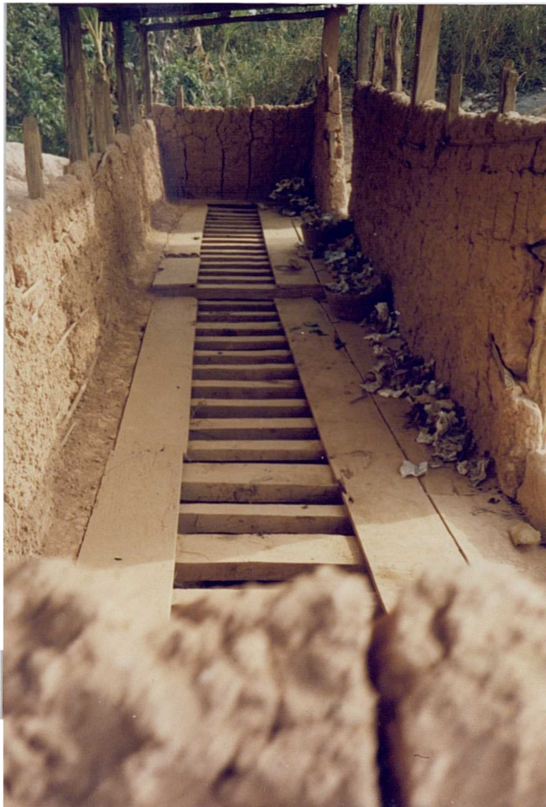
PLATE 7.20 INTERNAL ARRANGEMENT OF TRADITIONAL PIT LATRINE _ NOTE ANAL CLEANSING MATERIAL
