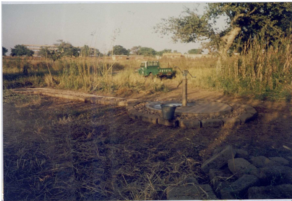
PLATE 7.7 MOYNO PUMP INSTALLATION WITH ANIMAL WATER TROUGH
