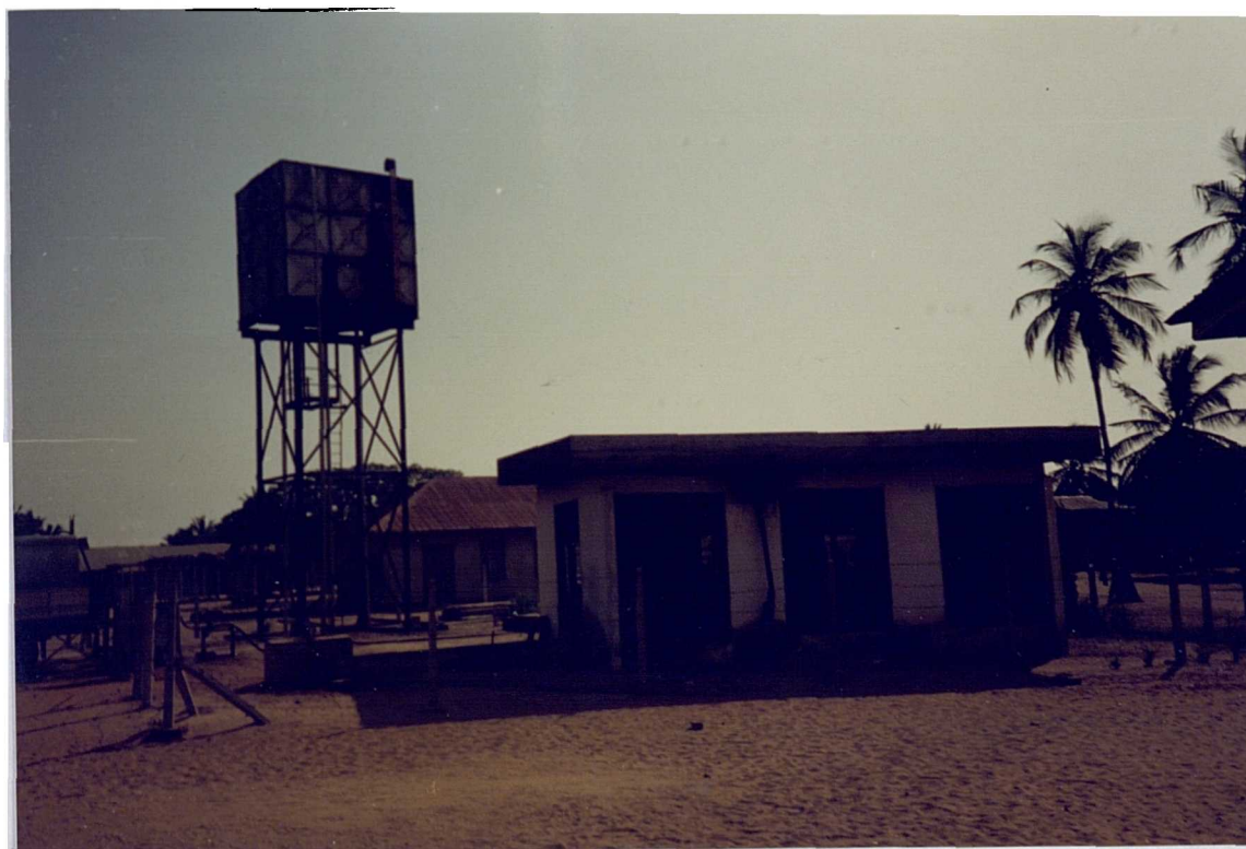
PLATE 7.4 BOREHOLE SCHEME WITH GENERATOR ROOM, ELEVATED TANK AND BOREHOLE COVERED IN CONCRETE CHAMBER
