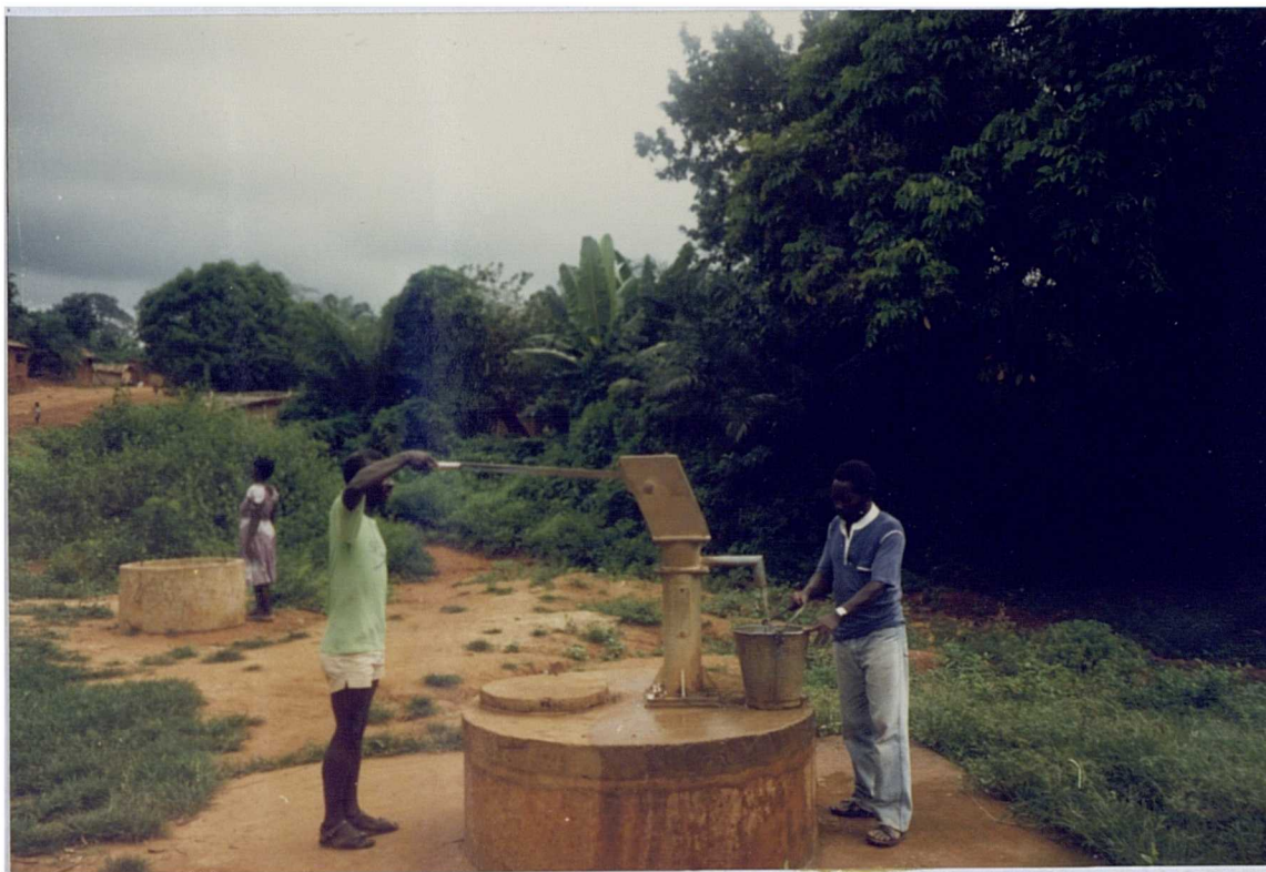
PLATE 7.11 INDIA MK 2 PUMP INSTALLED ON HAND DUG WELL - NOTE HATCH ON WELL COVER
