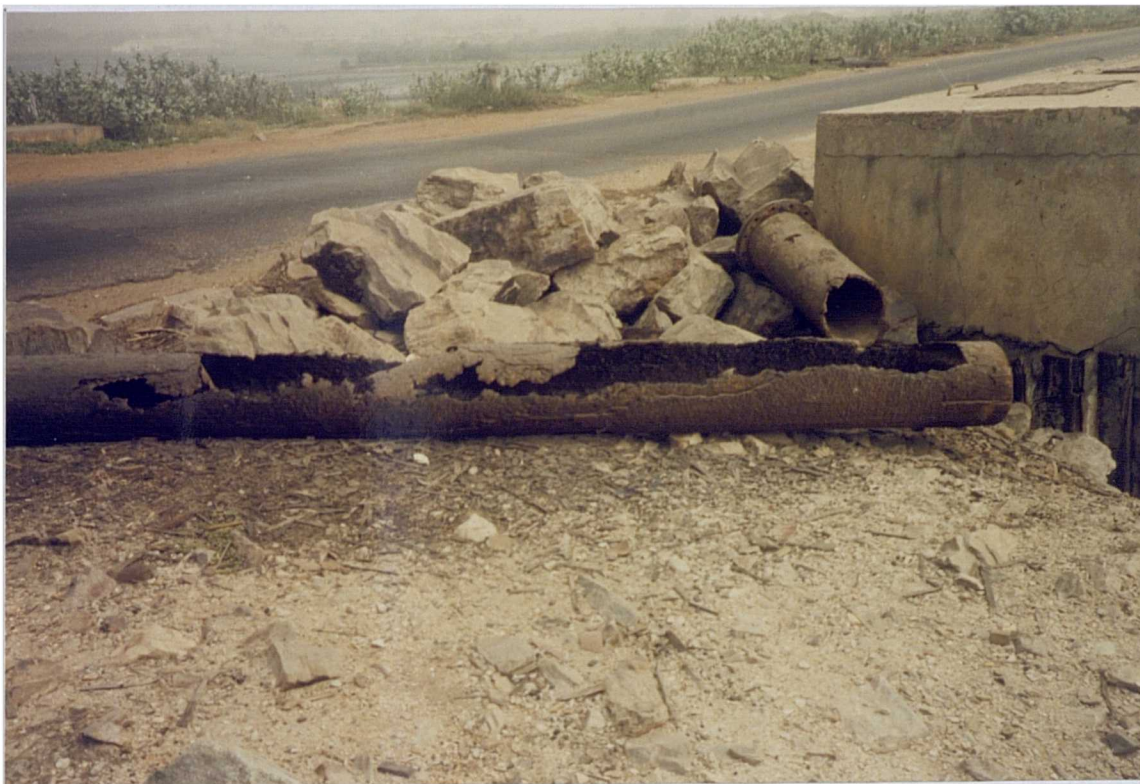
PLATE 7.13 CORRODED DISUSED STEEL SEWAGE OUTFALL
