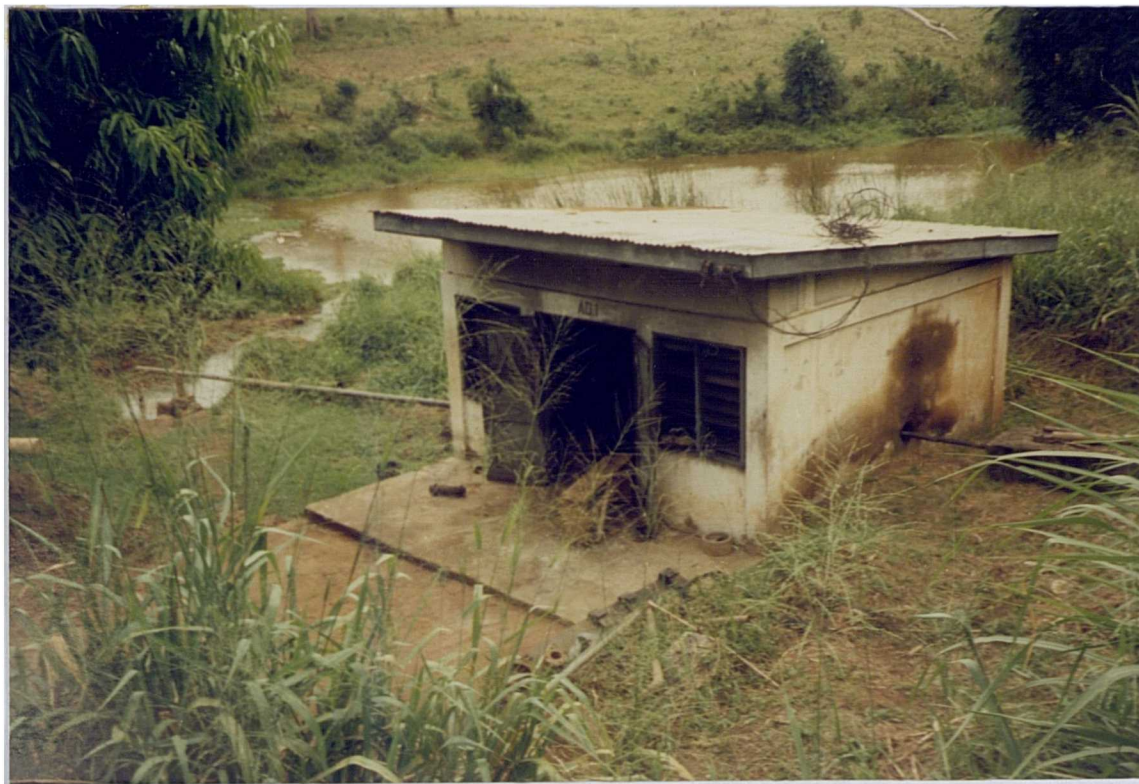
PLATE 7.5 RIVER INTAKE WITH PUMP AND GENERATOR ROOM
