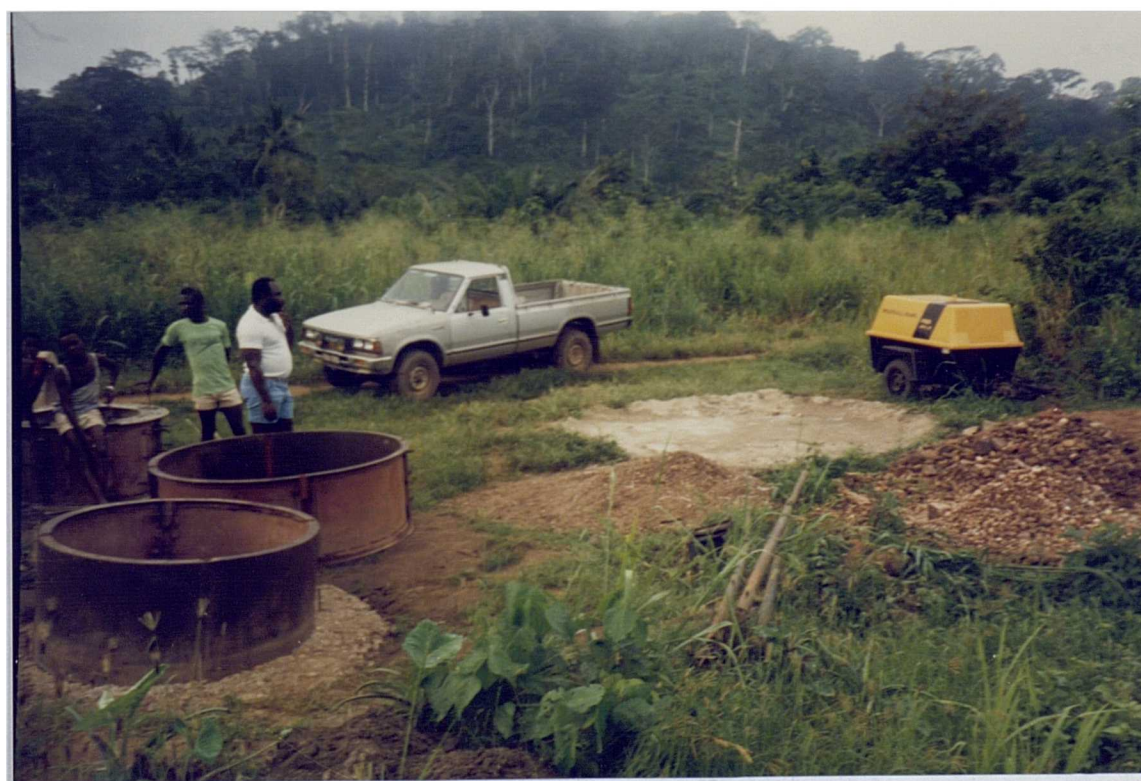
PLATE 7.12 STEEL FORMS, AIR COMPRESSOR, PROJECT VEHICLE AT A NEW WELL SITE
