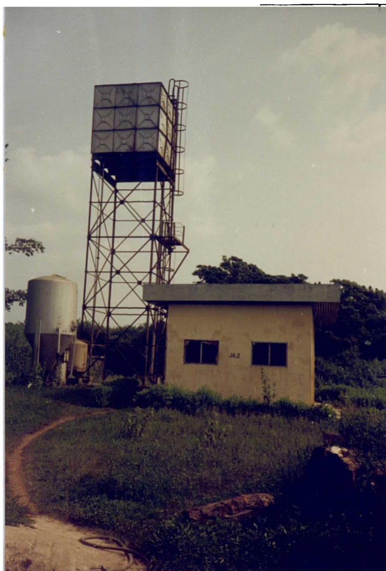
PLATE 7.6 PACKAGE PLANT WITH TREATMENT ROOM
