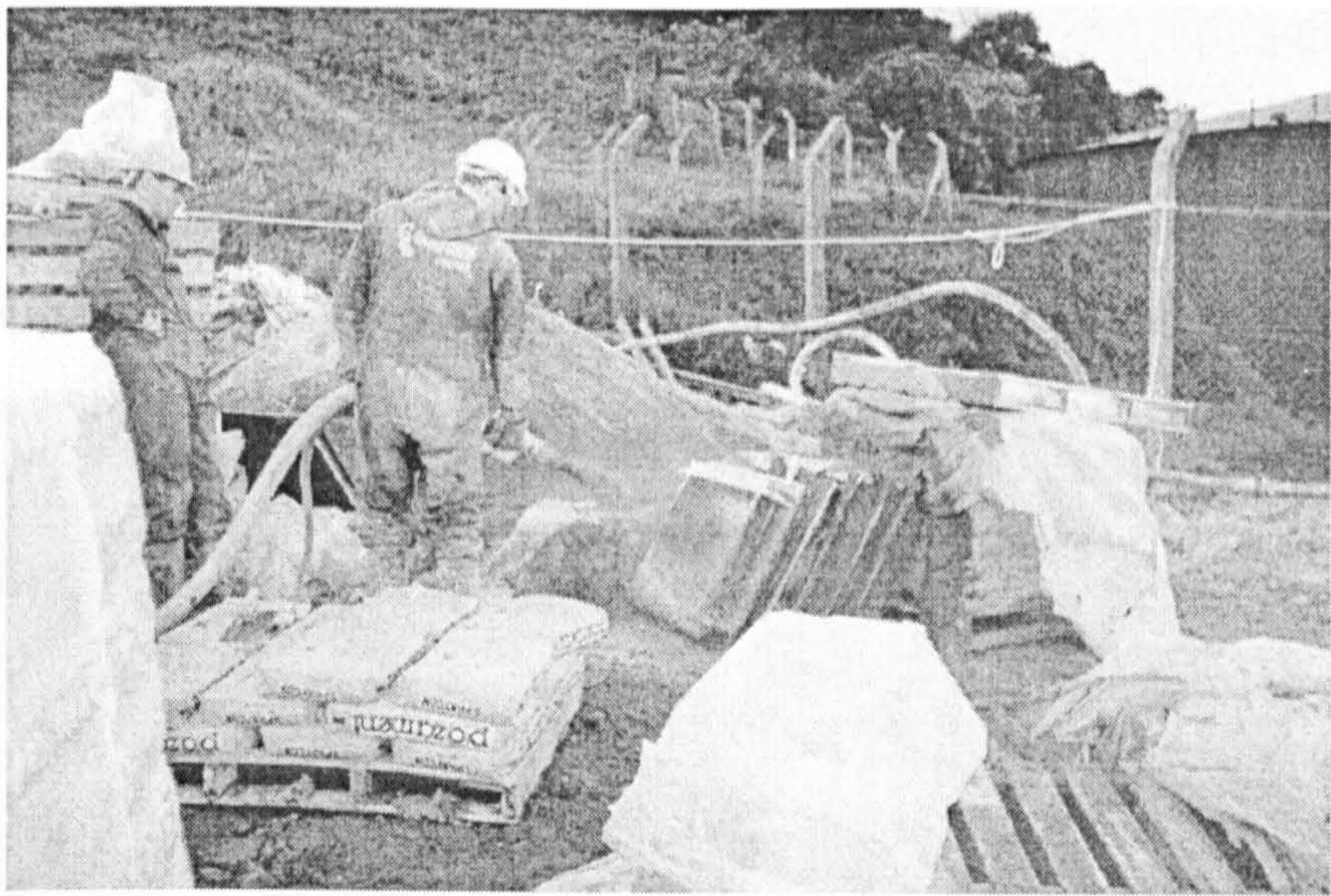
Figure 5.4 A test panel being sprayed during the spraying trial.
