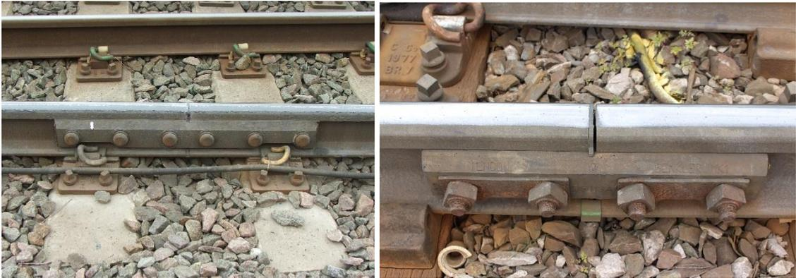
Figure 2.12 (i) A glued 6-bolt IRJ and (ii) a dry 4-bolt IRJ
