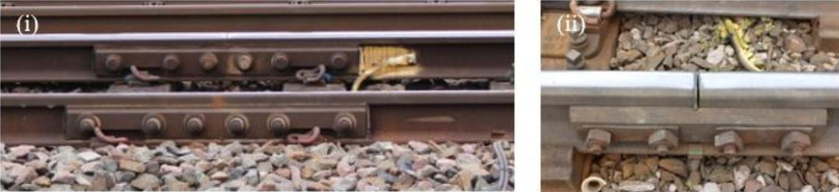
Figure 1.7 (i) 6-bolt and (ii) 4-bolt rail joints in UK site 2015 (Author’s personal collection)
