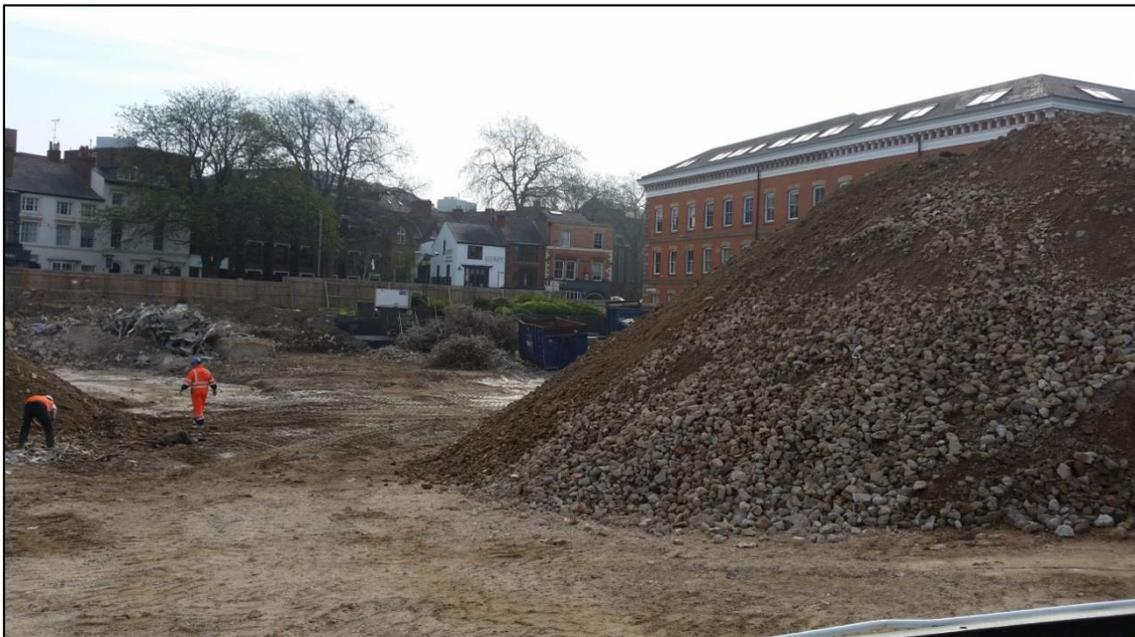
**Figure 4.5 Coarse CCA obtained from demolition site in Leicester, UK**
