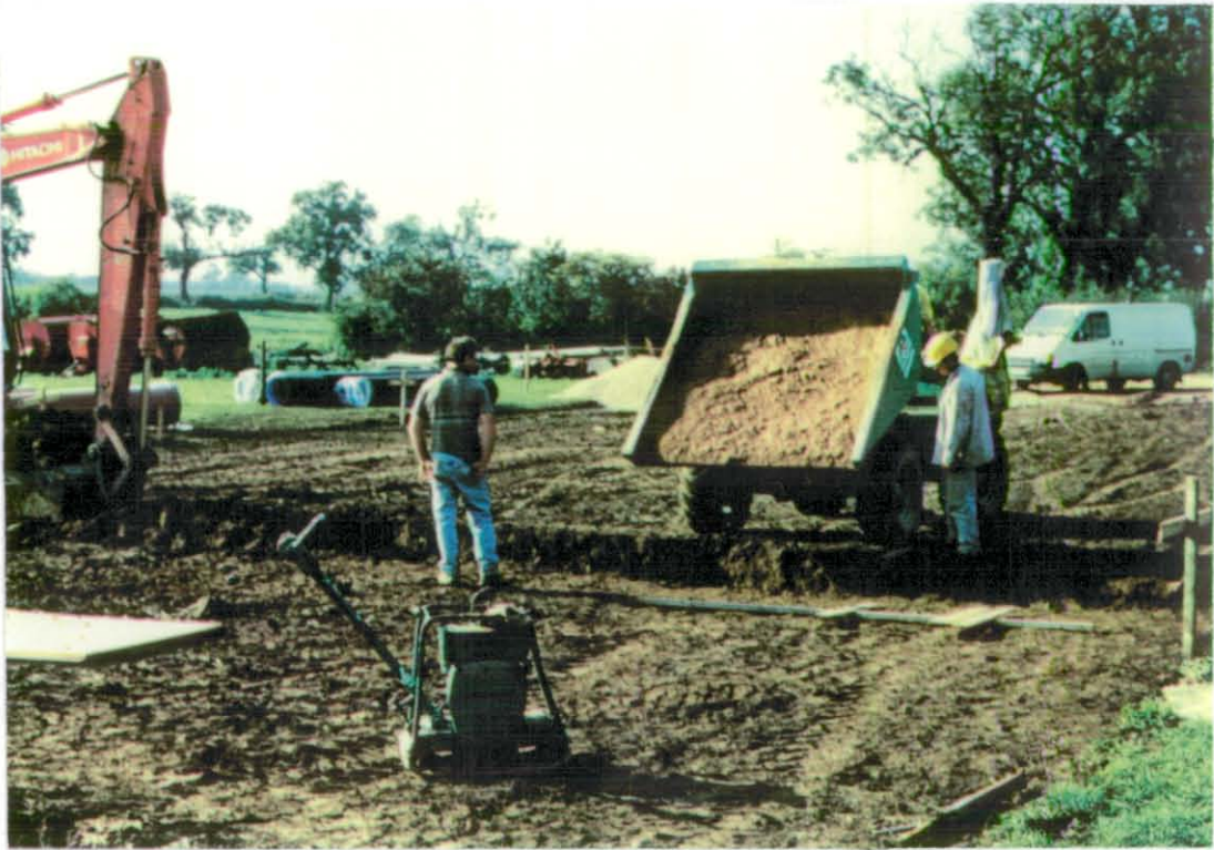
Figure 4.8. Placing of Surround Material.
