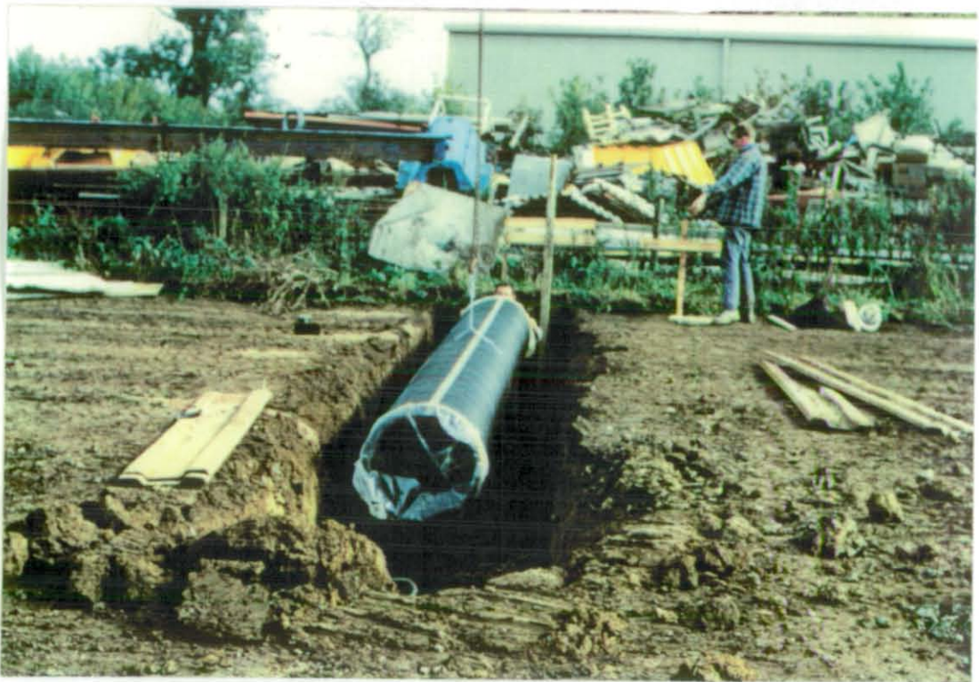
Figure 4.7. Lowering of Pipe into Trench.
