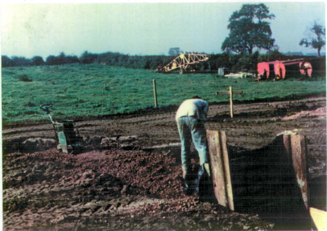
Figure 4.9. Placing of Trench Fill Material.
