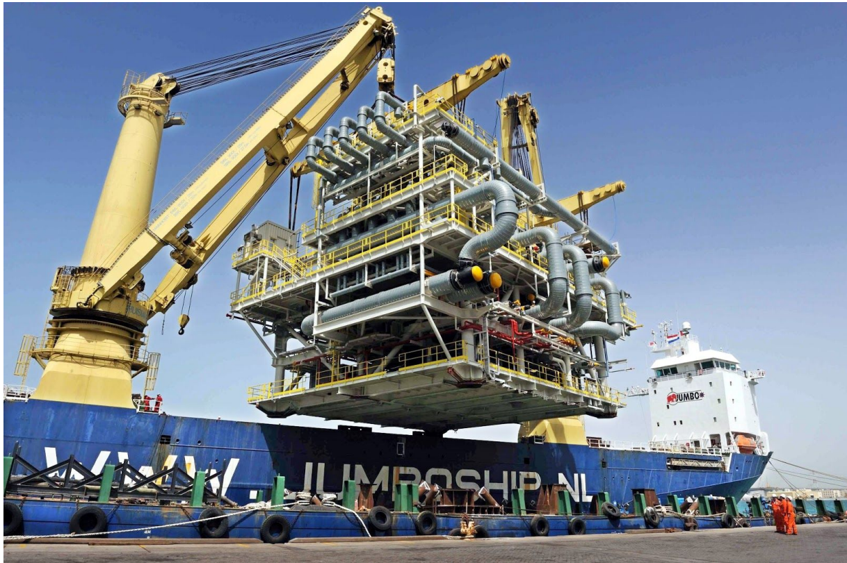
Figure 1. Module unloading at liquefied natural gas loading facility at ??? for Qatargas (courtesy Fluor Construction and Fabrication, Amsterdam)
